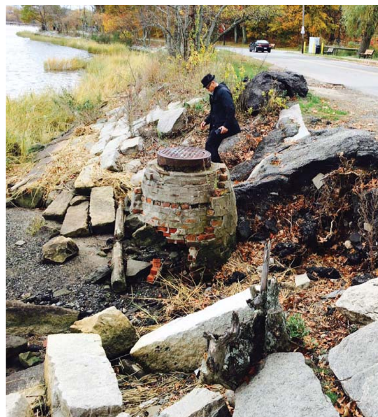
Existing Conditions: River Road stormwater outfall "chute" (top) and riverbank condition (bottom)
